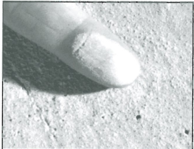
Dusting concrete surface
