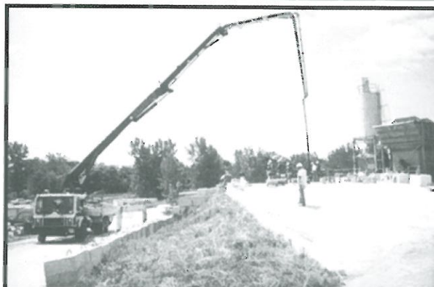
Figure 1: A vertical pump boom configuration can result in loss of entrained air in concrete
