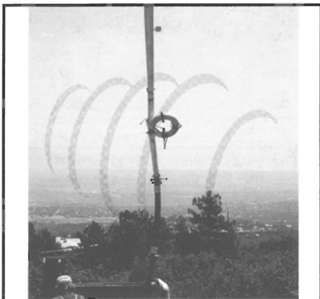
Figure 2: Loop in pump boom
